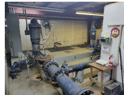
Existing status of Grainger Springs Pump House
